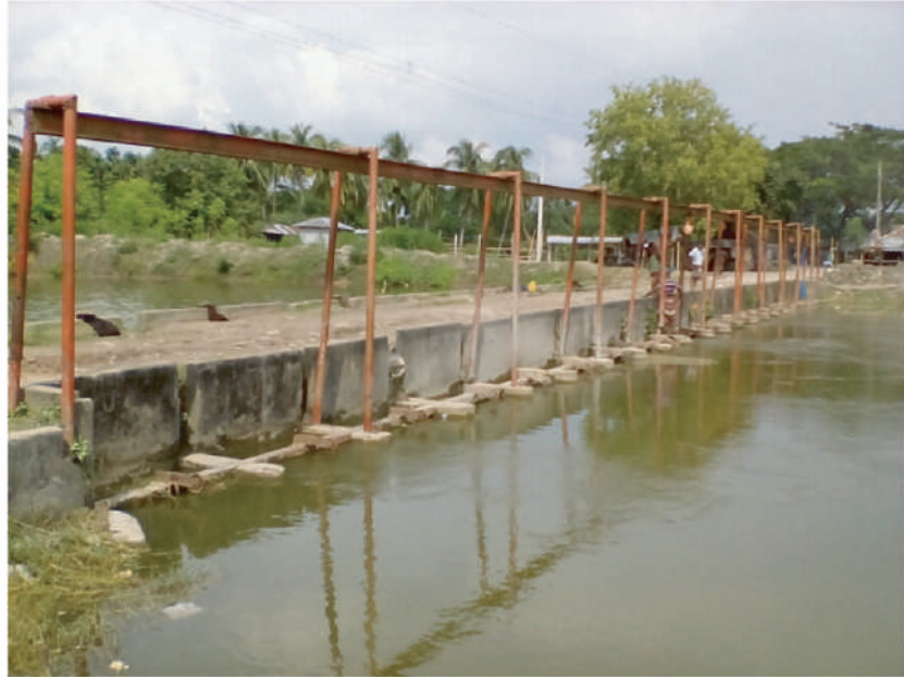
Bhabodah Sluice gate
