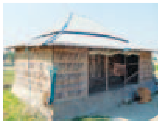
Picture 4-35: Traditional house in project area
