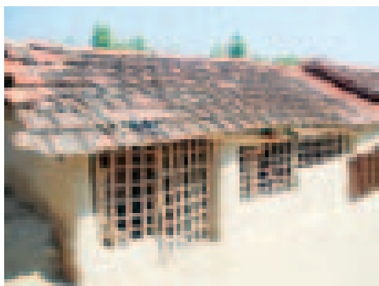
Picture 4-34: Traditional house in project area
